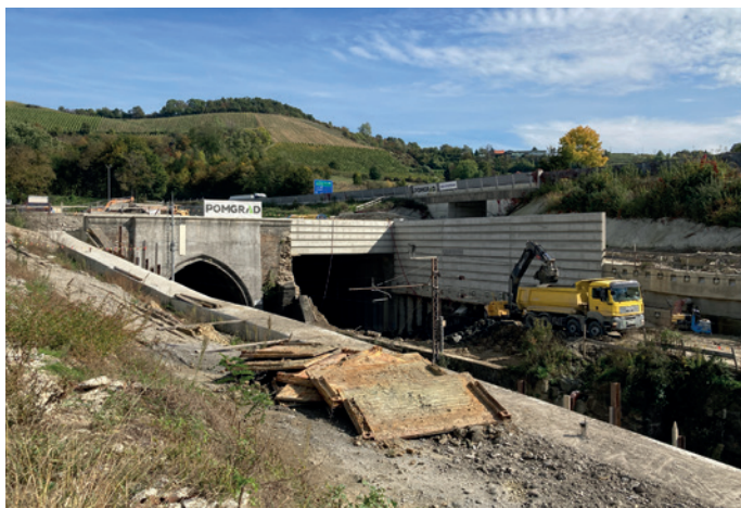
2021, portal starega in novega predora Pekel na J strani
